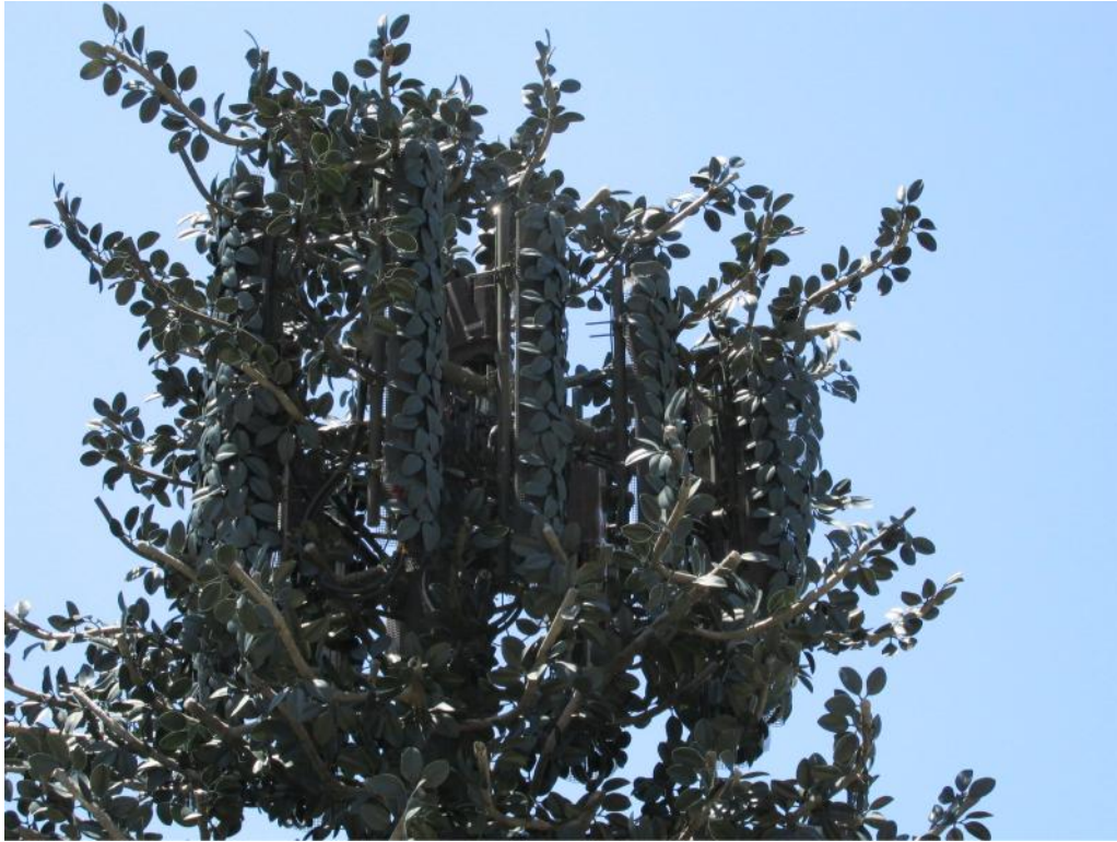
Figure 4: Verizon Wireless Gamma Sector Antennas #9 through #12
