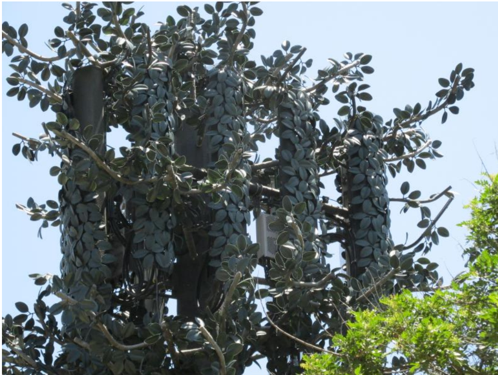
Figure 3: Verizon Wireless Beta Sector Antennas #5 through #8
