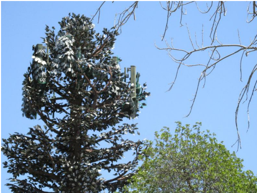
Figure 17: Sprint Decommission iDEN Antennas #34 through #36
