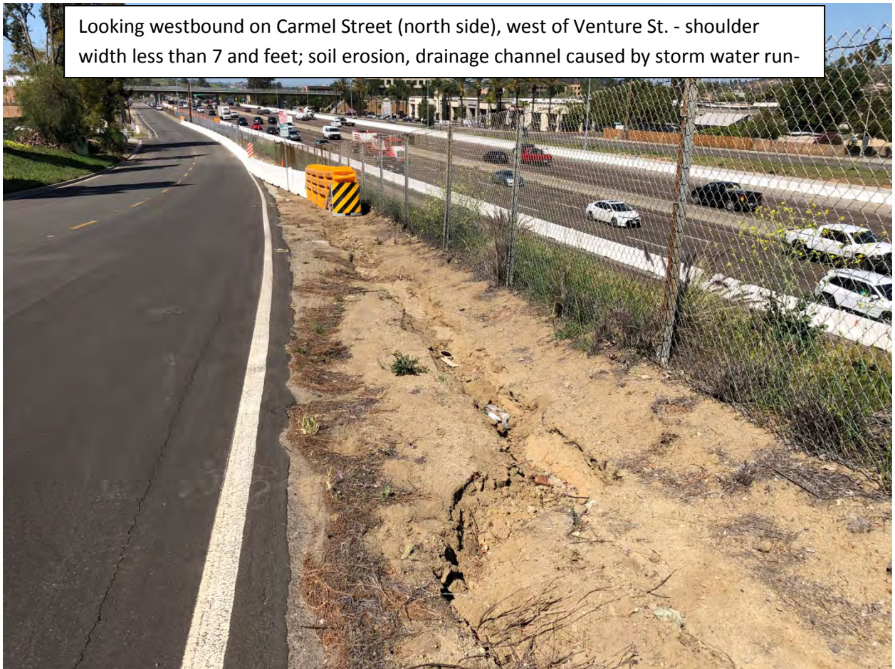
Looking eastbound on Carmel Street (north side), west of Venture St. - shoulder width less than 7 and feet; soil erosion, drainage channels/gullies caused by storm water
