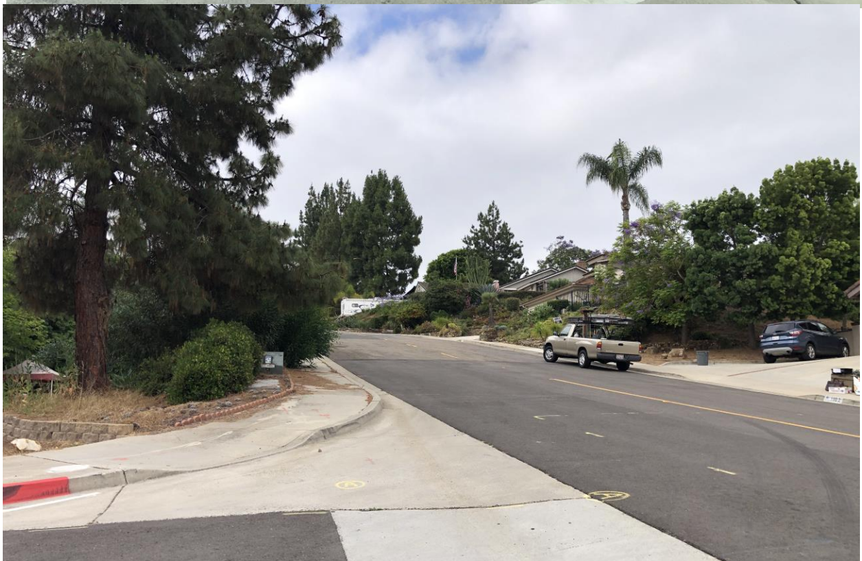
Looking southbound on La Sombra Drive from Quail Hill Drive intersection Recommend tree/vegetation trimming or removal to improve line of sight around roadway curve
