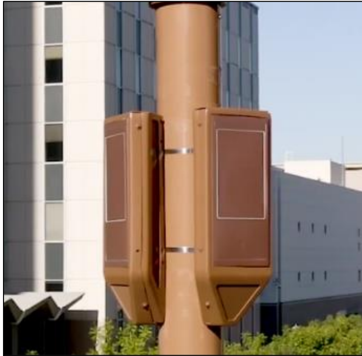
Figure 2: 5G mmWave antenna/cable shrouds
