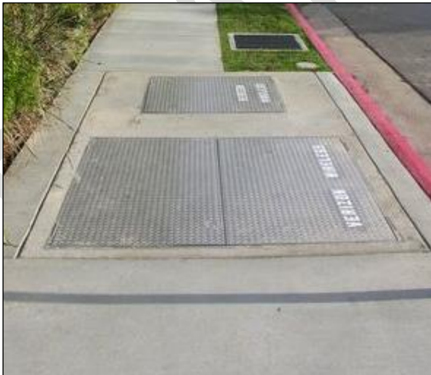
Figure 8: Flush-to-grade underground equipment vault
