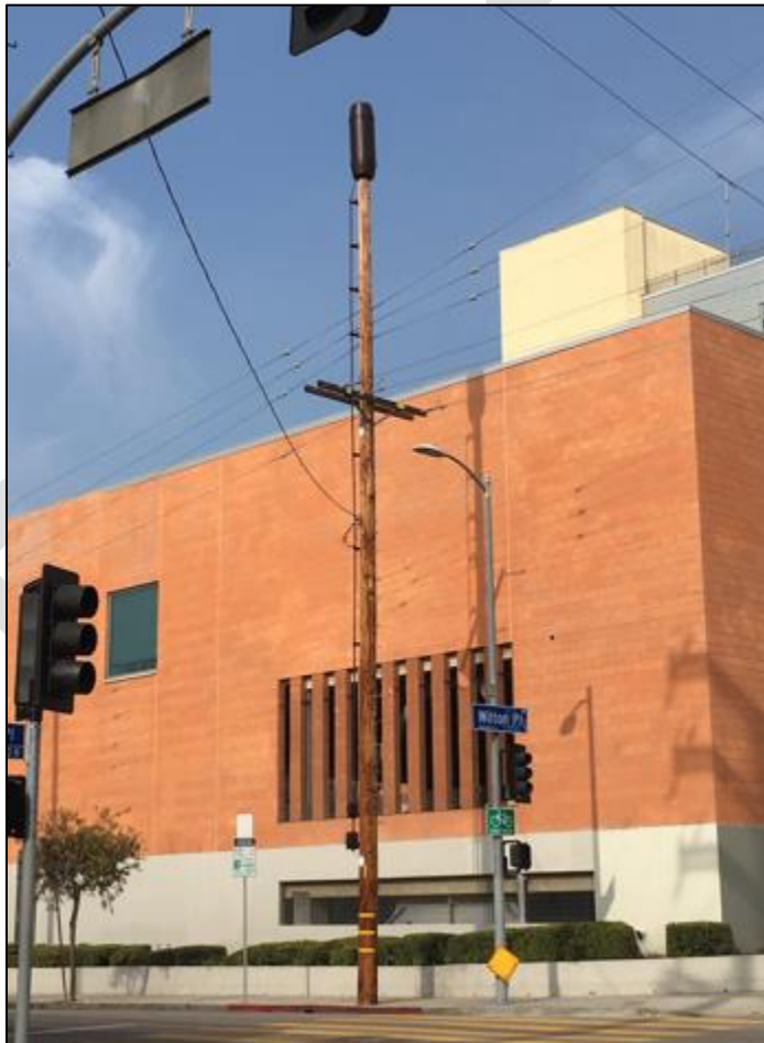
Figure 5: Pole-top antenna on a wood utility pole
