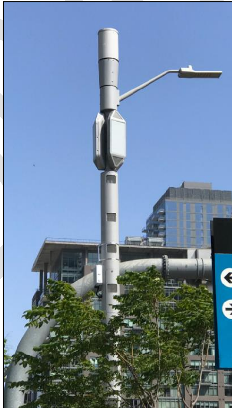
Figure 3: 4G/5G configuration with antenna/cable shrouds
