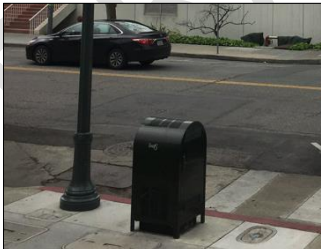
Figure 7: Ground-mounted accessory equipment stealth concealed as a mailbox.
