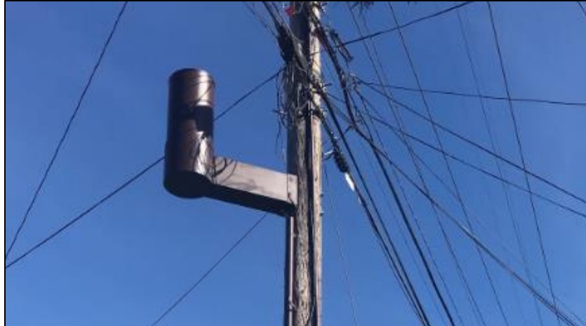
Figure 4: Shrouded, side-mounted antenna on wood utility pole to comply with CPUC horizontal separation requirements
