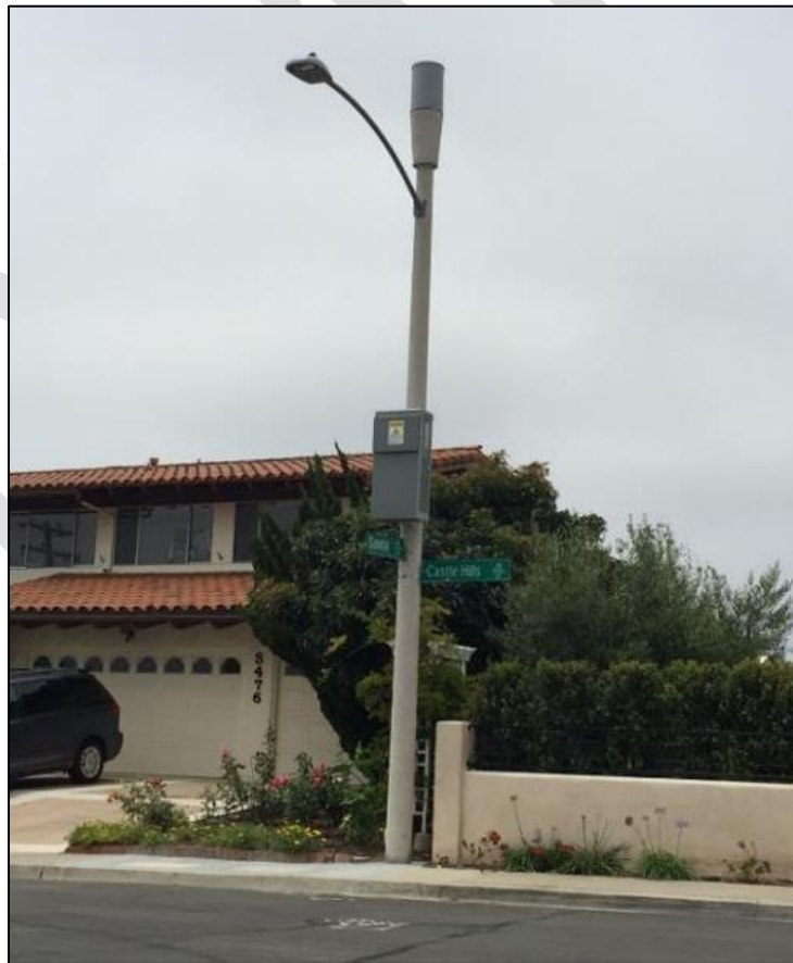
Figure 1: Pole-top antenna stealth concealed within a single shroud (or radome) with a tapered cable shroud.
