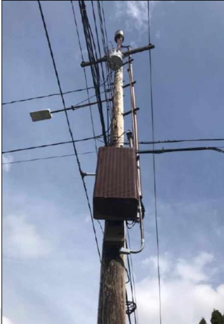
Figure 4: Pole-mounted accessory equipment shroud on a wood utility pole
