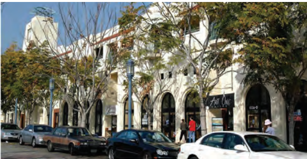
Image 20.225-14 A, B, C Storefront Conditions
