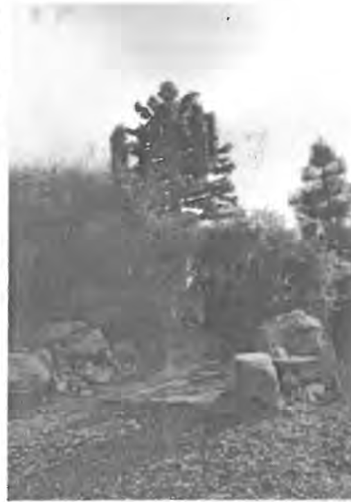
Picture taken in January of 2014 after antenna retrofit.
